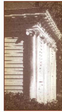
Becker College's pump house.
