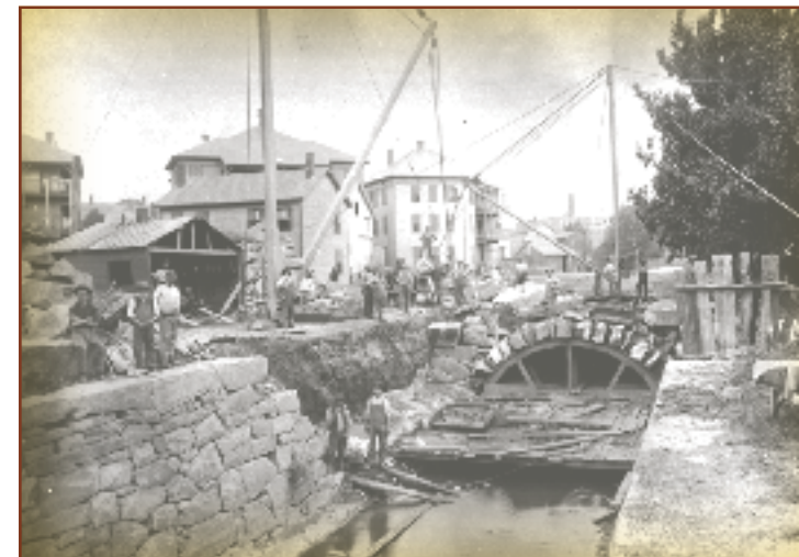
When the Blackstone Canal Company folded, parts of the abandoned trench deteriorated into rank open sewers. During the 1890s, they were sensibly integrated into Worcester’s underground waste water system. Dressed granite blocks from the 13-foot walls of the 82-foot long locks were sold and carted away to become parts of new buildings. During deep excavations, the city’s highway department even now sometimes uncovers the canal.
