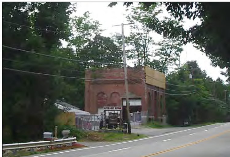
Harmony Trolley Power Station
