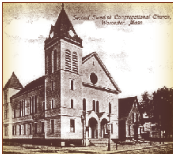
The First Swedish Congregational Church built a Chapel for the villagers in 1891 on Greenwood Street. Between 1899 and 1901, Village Congregationalists built the Second Swedish Congregational Church (shown c 1910), beside the old Chapel on Greenwood Street.
